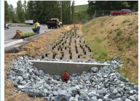
Logistics Bioretention Swale
